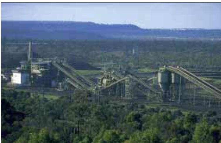
Coal from the mine is washed and sized in the preparation plant before being loaded for transport by rail.
